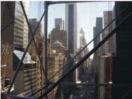
Construction constraints were many for this tight site in Manhattan.
